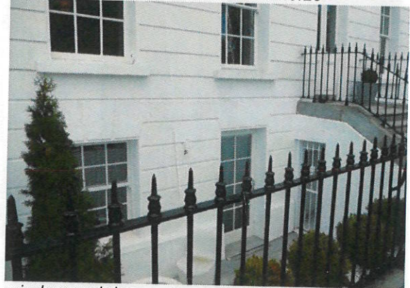
window and door at basement of no.27
