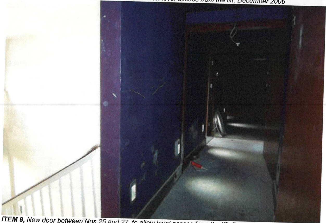
ITEM 9, New door between Nos.25 and 27, to allow level access from the lift, December 2006
