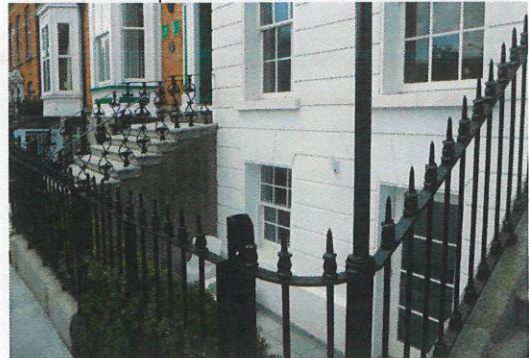
window and door at basement of no.29
