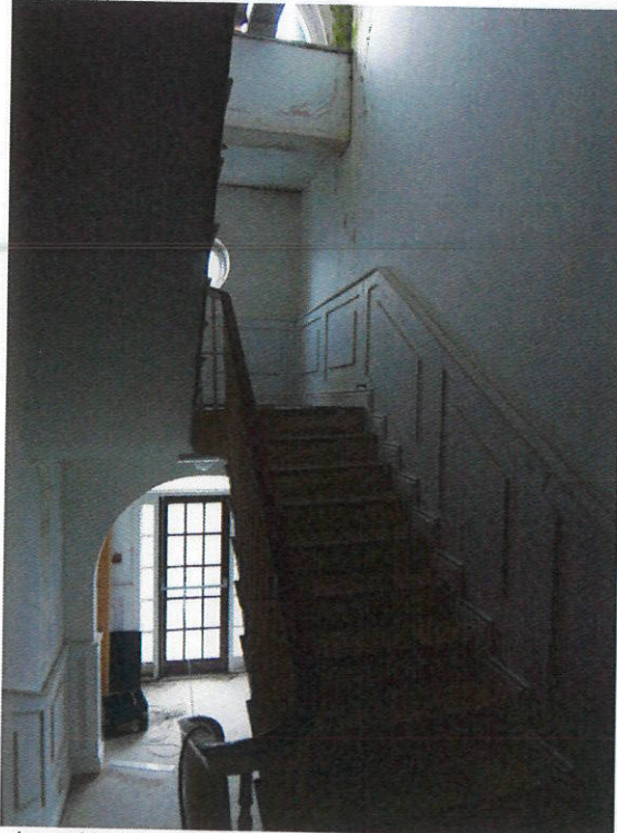
view of half landing in no.27, which links to no.25
