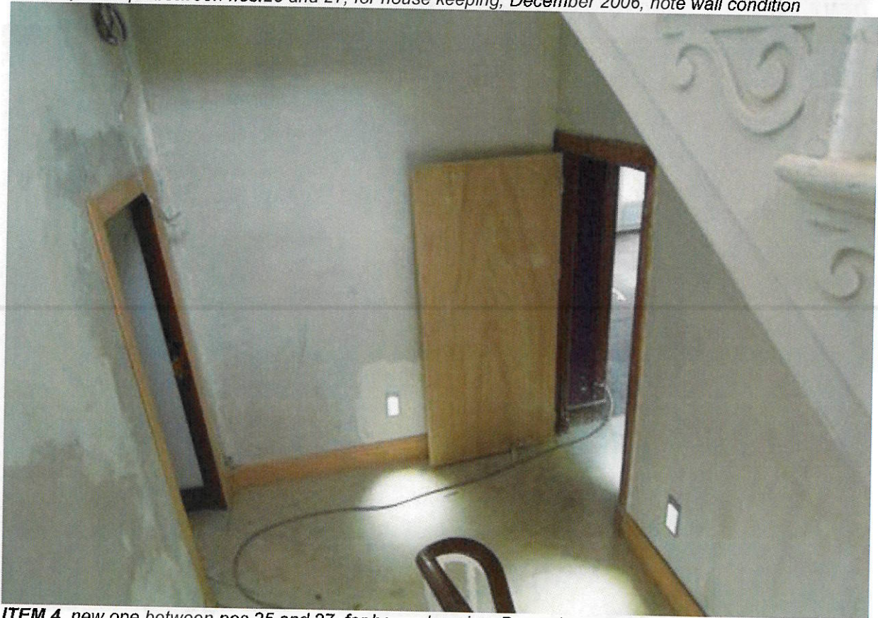
ITEM 4 , new ope between nos.25 and 27, for house keeping, December 2007, left hand side
