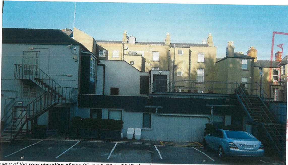
view of the rear elevation of nos.25, 27 & 29 in 2017 showing the revised escape stairs and the roofed portions, which are located over the 20 th century single-storey part of the building
