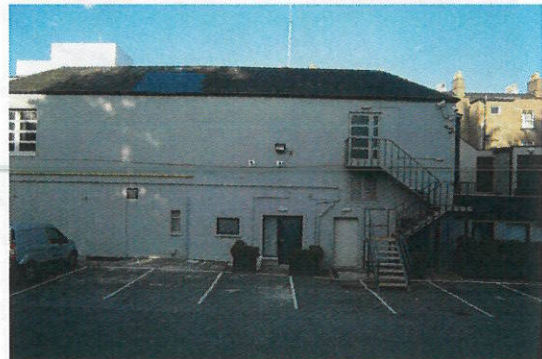
rear elevation of the function room
