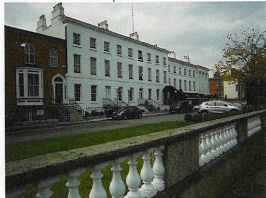
front elevation of Nos.19 – 29, Morehampton Road
