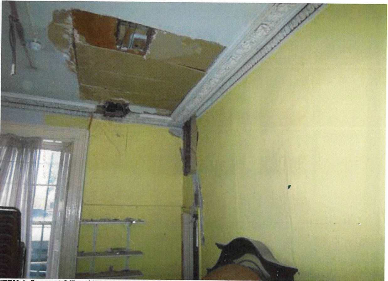
ITEM 1, Banquet Office, No.26, December 2006, showing existing ceiling
