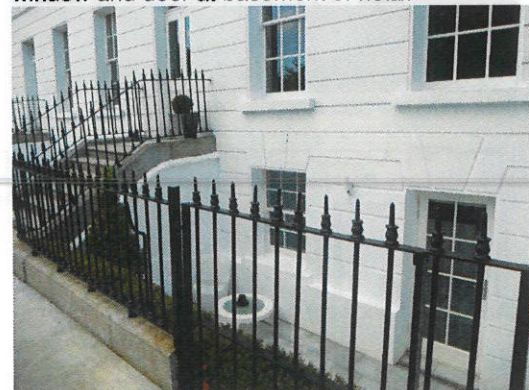
window and door at basement of no.25
