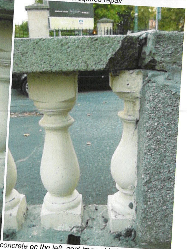
view of the second section of balustrading that was not damaged, but that requires repair
