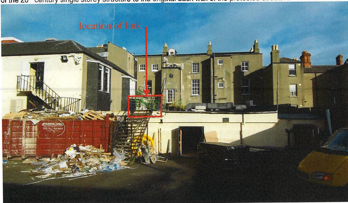
view of the rear elevation of nos.25, 27 & 29 in 2007-area of first floor link shown in red
