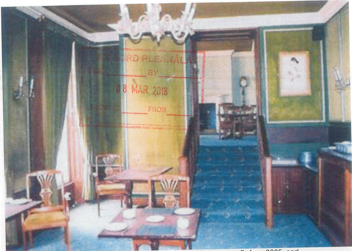
ITEM 5 , Relocation of modern stairs between Nos.23 and 25, to rear wall, June 2005, and ITEM 6 , Alteration of former restaurant to bedrooms, Nos.21, 23 and 25, view from 23 to 25 June 2005 Note modern cornices and modern panelling
