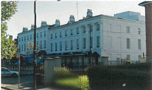
front elevation, looking southwards
