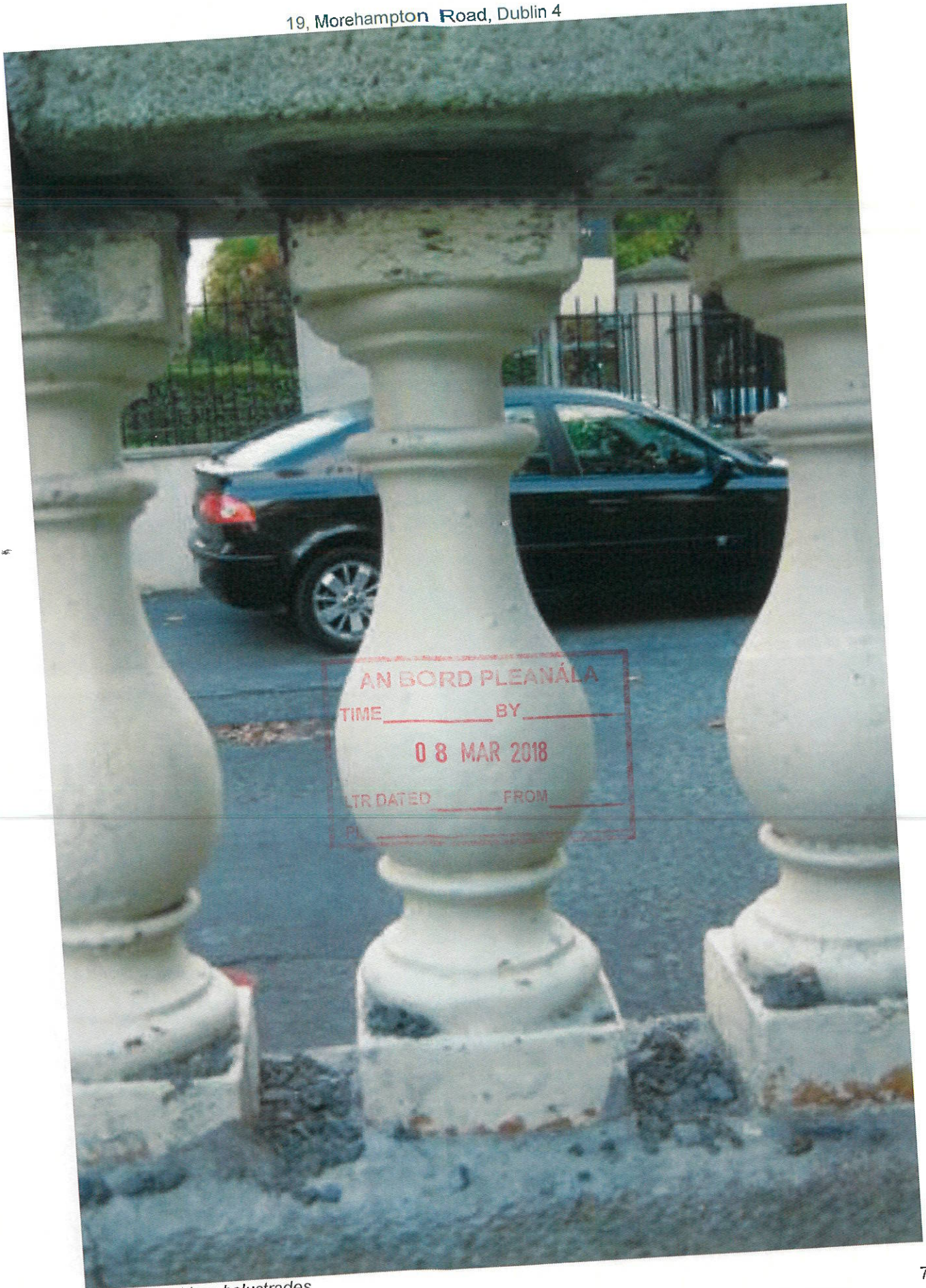
detail of cast iron balustrades
