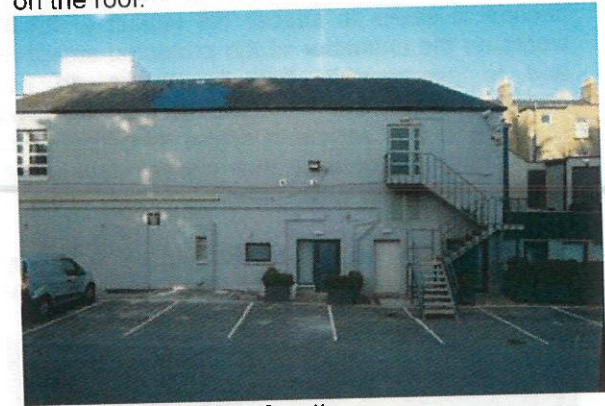
rear elevation of the function room
