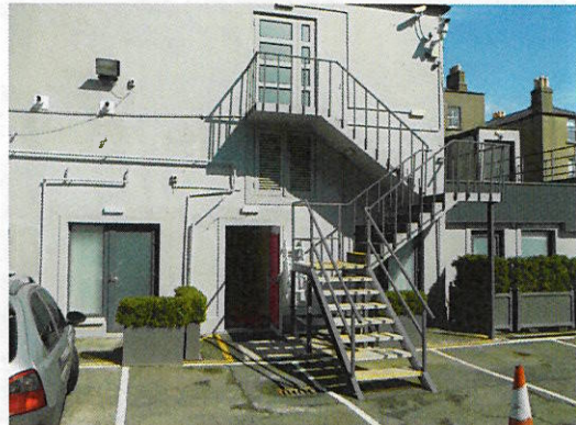
view of the last leg of the fire escape
