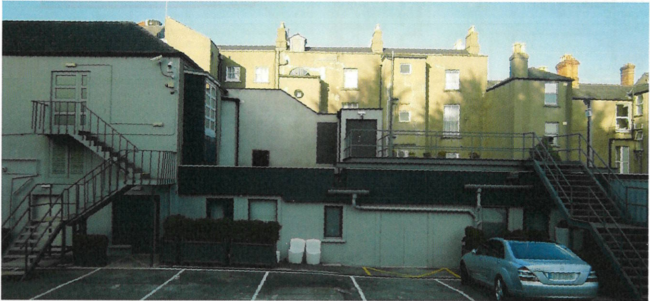
View of the altered fire escapes to the rear of the 20 th /21 st century buildings
