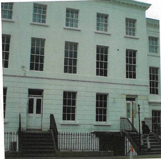
no.25 in 2008 (during refurbishment)
