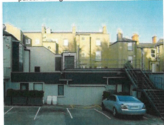
view of the fire escape route and stairs to the right
