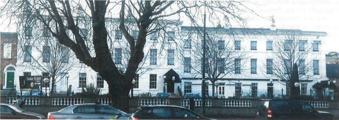
view of the buildings in 2017 showing the effect of the works for which the Section 5 application is being sought
