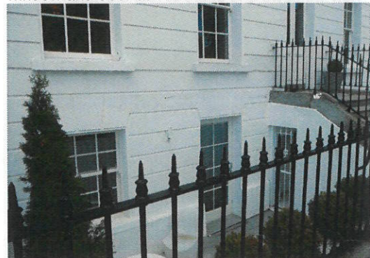
window and door at basement of no.27
