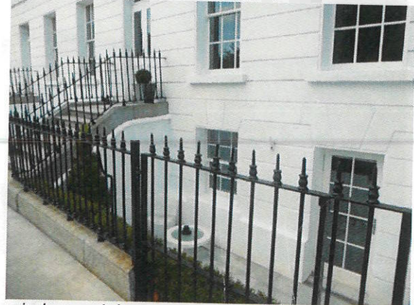
window and door at basement of no.25
