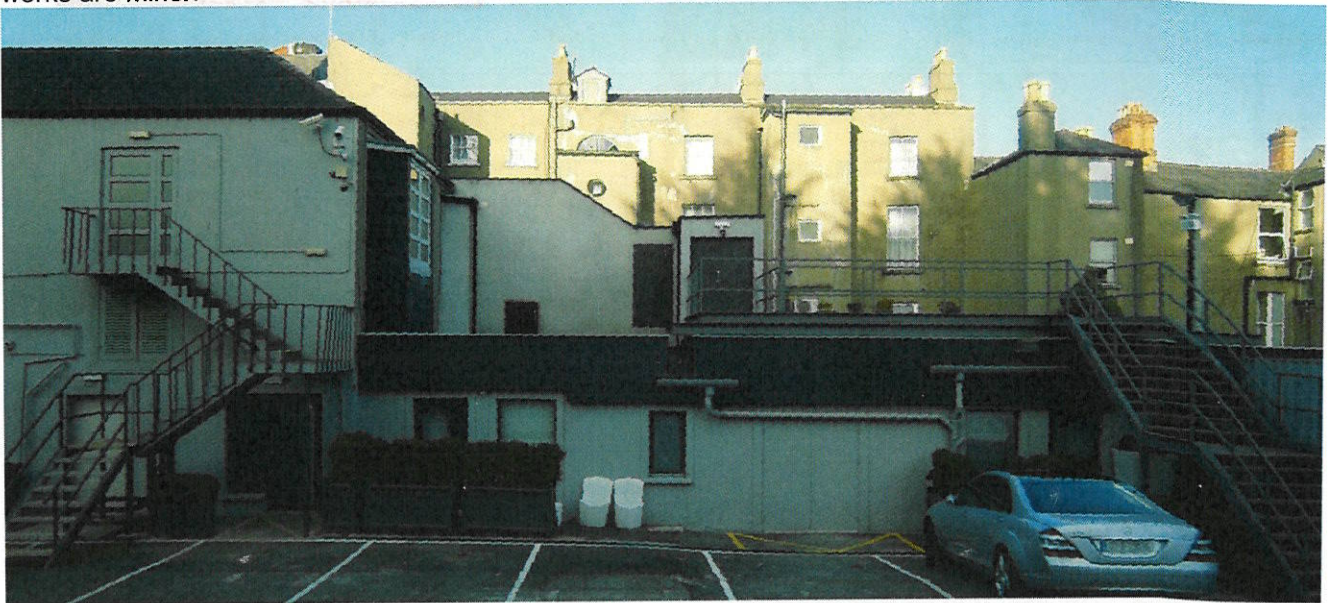
View of the altered fire escapes to the rear of the 20 th /21 st century buildings
