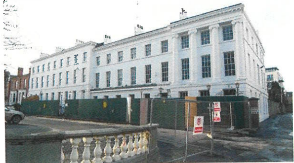
front elevation of Nos.19 – 29, Morehampton Road
