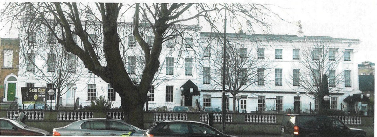
view of the terrace in 2017, with landscaped area outside no.21 Morehampton Road to the right hand side
