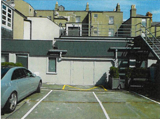
new windows and doors in rear elevation
