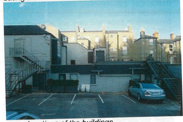
rear elevations of the buildings
