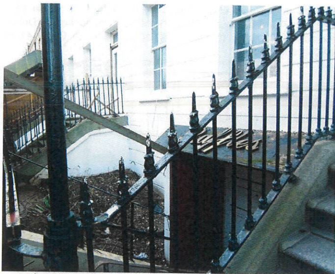
no.25 in 2008 (during refurbishment)
