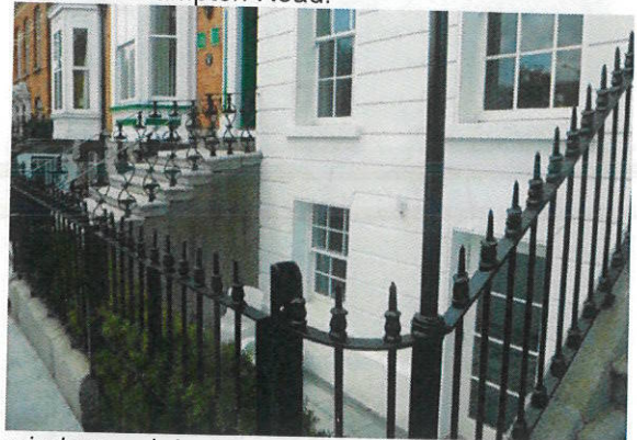
window and door at basement of no.29
